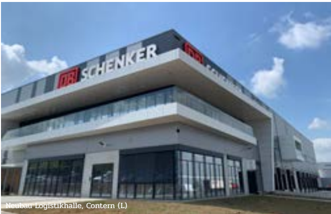
Neubau Logistikhalle, Contern (L)
